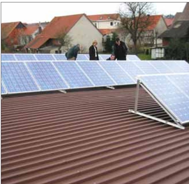
Photo 2. PV system being installed
